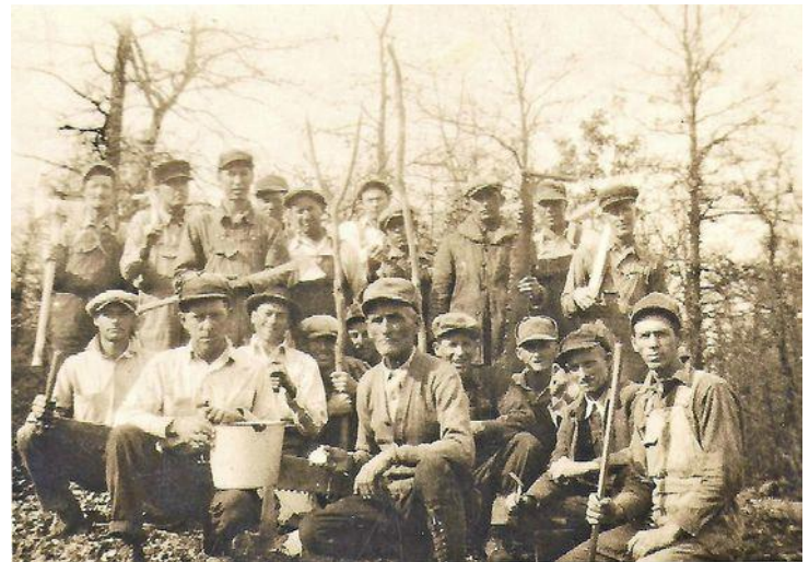
Men on a work crew clearing land for the making of Lake Murray, In Carter County, Oklahoma
